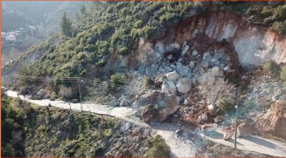
Rockfalls were generated by the earthquake along a hill adjacent to Bektasli village, causing damage to buildings and 49 fatalities. Boulders were detached from the mountain and then rolled and crushed one-story houses in the village resulting in total destruction.
