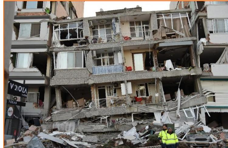
In several cases, although the structures have not completely collapsed, their load-bearing system has suffered significant damage that is considered beyond repair.
