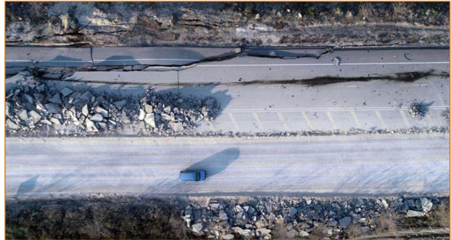
The Antakya Demirözü highway, the road connecting Antakya to Reyhanlı district suffered heavy damage by the severe earthquake ground motion. The road was heavily cracked for a length of about 1 km.
