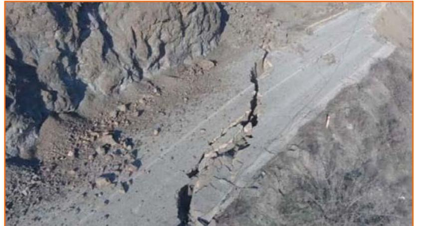
Part of the road leading from Kahramanmaraş to Malatya collapsed leaving only two of the four road lanes in place. In some places the landslide was 8 meters long. In addition, rockfalls were generated from adjacent slopes. Source: <https://www.cnnturk.com/turkiye/depremin-otoyollardaki-tahribati-hem-yarildi-hem-coktu?page=2>
