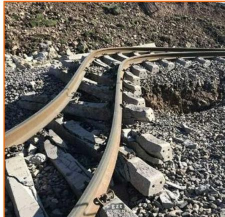
Railway tracks were heavily deformed due to the surface ruptures. They were restored few days after the occurrence of the earthquake.
