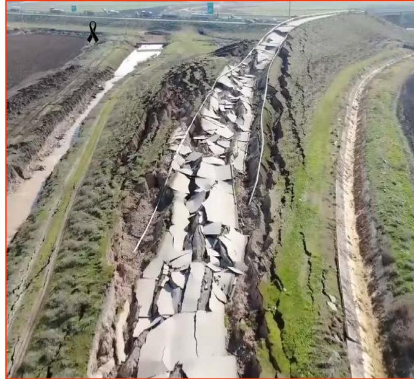
The collapse of the road to the village of Koseli, which passes over the Adiyaman-Sanlıurfa-Gaziantep Highway is attributed to earthquake-induced lateral spreading. The huge ground cracks are representative of the earthquake magnitude.
