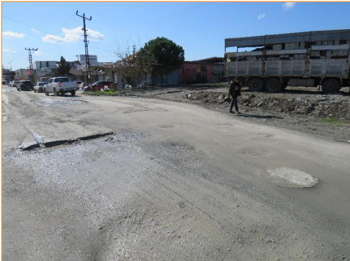
Liquefaction phenomena were triggered in several parts of the affected area. They comprised ejection of liquefied material from cracks, which covered large parts of the road and affected adjacent structures and infrastructures.
