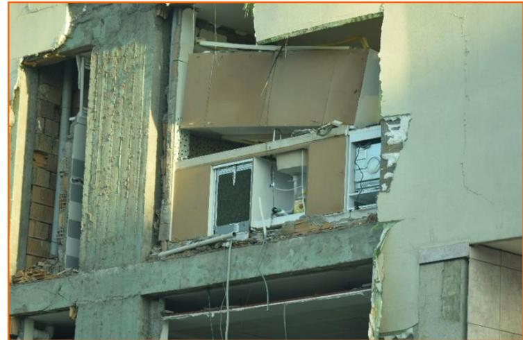
The load-bearing system of many buildings' has not suffered significant damage, in contrast to the external infill masonry, as well as some (internal) partition walls, which have -in some cases- completely collapsed.
