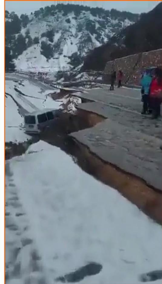
A lateral spreading failure on a river bank affected the road between Adana and Gaziantep.
