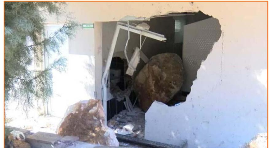
In the Bektaşlı village of the Kırıkhan district of Hatay, the rocks that broke off the mountain due to the effect of the earthquake rolled and fell on the one-story houses. Source:
