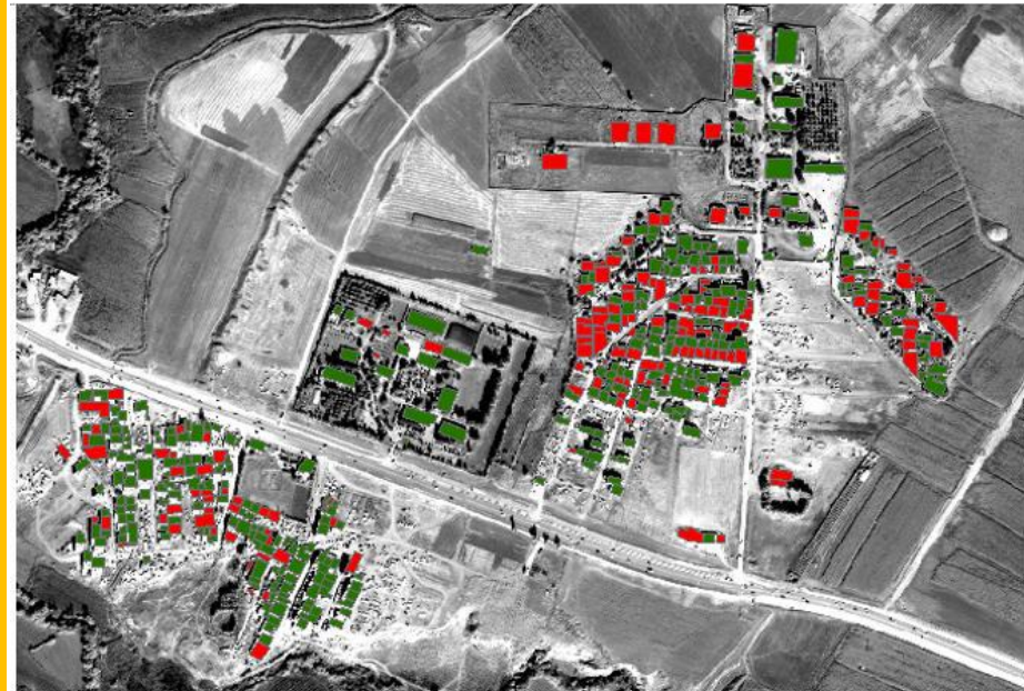
ANN's damage mapping using only post_event damage map
