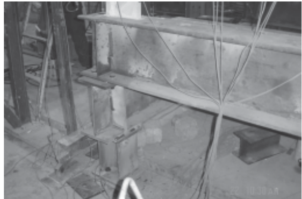
b) Locking the Foundation to the Strong Floor
