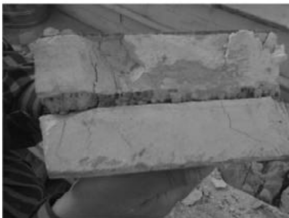
Experimental Cracks and Failure
