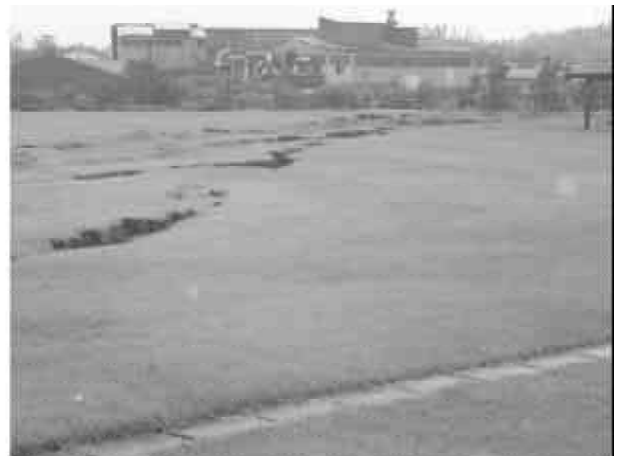
Figure 12. Damage to sheet pile type quay wall with tie rods in Kashiwazaki fishery port due to settlement where the evidence for liquefaction was also found.
