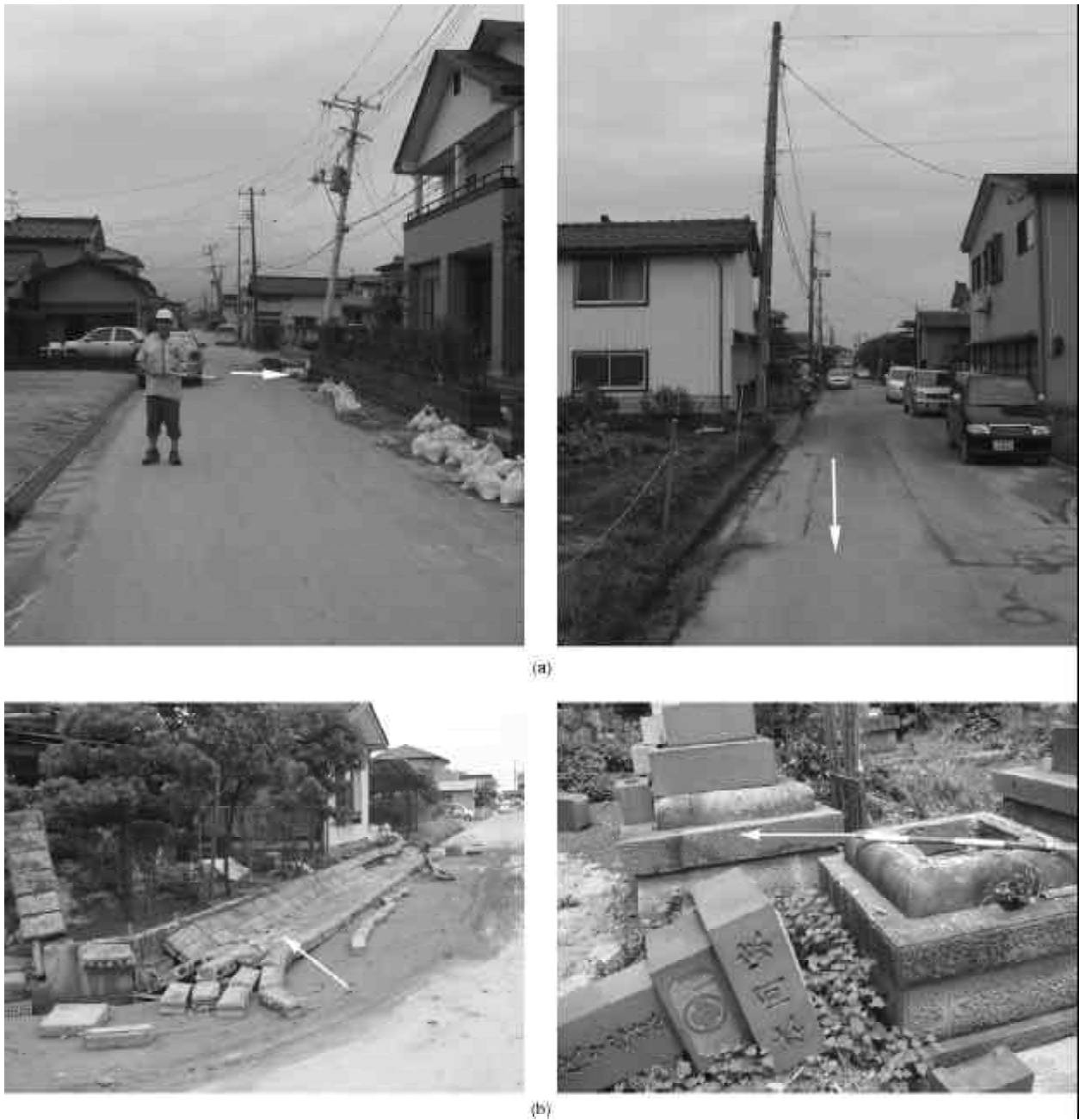
Figure 20. Evidence for directional damage (the arrows show the north side); (a) electrical poles directed in EW direction displaced more in comparison with those directed almost in NS direction at Matsunami 2; (b) The toppling direction of the concrete block fences and tomb stones in Kashiwazaki area, see Figure (21).
