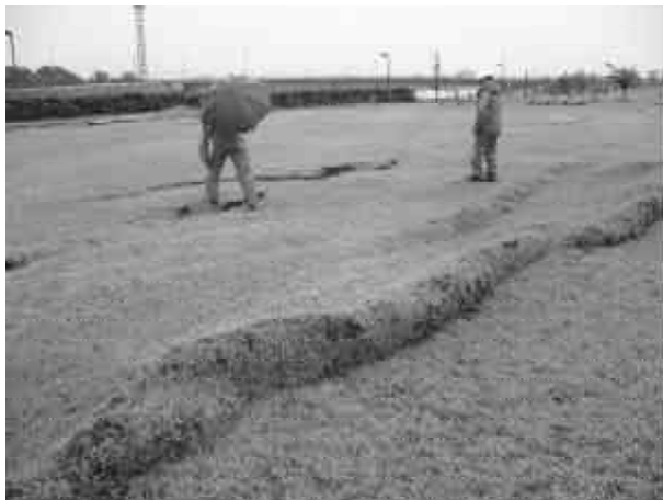
Figure 12. Damage to sheet pile type quay wall with tie rods in Kashiwazaki fishery port due to settlement where the evidence for liquefaction was also found.
