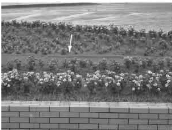
Figure 13. Large ground fissures due to liquefaction at the Sabaishigawa Kaishu-Kinen Park in Makhara-Kashiwazaki. The park was constructed on a sandbar along the Sabaishi river.
